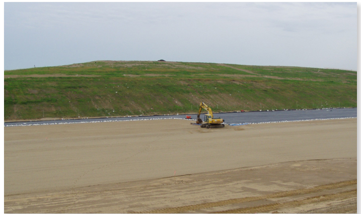
Michigan landfill in the process of cell construction.
