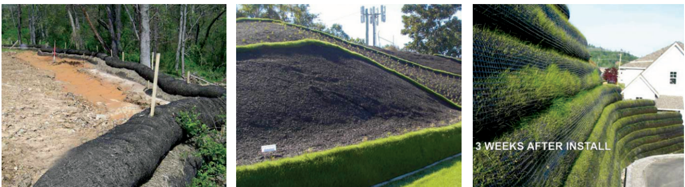
Figure 1-30: (Top) Sediment trap, (middle) Slope protection and erosion control blanket made from compost, (bottom) vegetated walls
