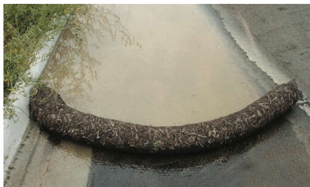
Figure 2-7: A tubular check dam made from compost intercepts stormwater to slow the flow velocity, while filtering sediment and pollutants. The water below the check dam is noticeably clearer and cleaner.
