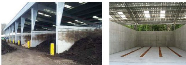
Figure A-5: Several facilities have been built using concrete bunkers to separate individual ASPs into rectangular-shaped piles by poured concrete or concrete block walls. The primary advantage of bunkers over piles is the vertical capacities gained by the separating walls compared to angle-of-repose individual piles.
