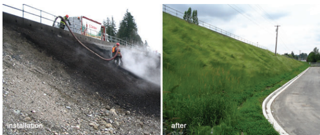
Figure 2-9: (left) Compost blanket being applied to steep roadway embankment, (right) Vegetation thriving after installation.
