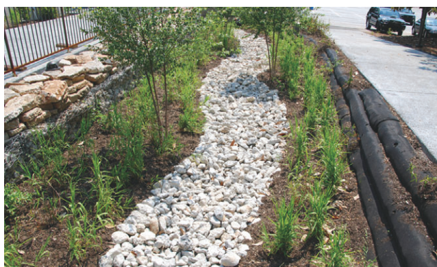
Figure 2-8: The above bioswale is a shallow landscape depression or channel used to convey, slow, and filter stormwater. Bioswale installations use organic matter and vegetation to create low-impact development (LID) that can serve as pre-treatment or post-treatment for stormwater containment systems while reducing runoff volume and peak flows.
