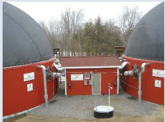
Figure C-3: Liquid AD System at dairy farm, Exeter, ME
