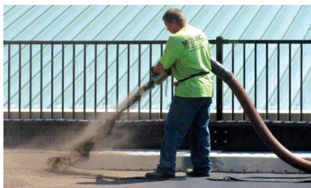
Figure 2-15: MCS Inc. worker installing growing media made from compost on green roof.
