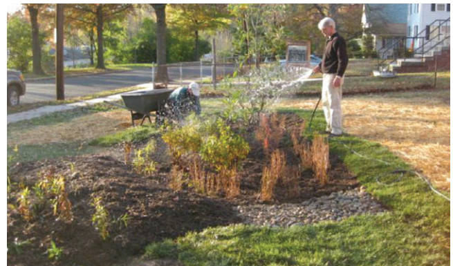
Figure 2-5: The Montgomery County, MD RainScapes Rewards Rebate program requires 3 inches of compost for its conservation landscape projects, incorporated to create a 6-12 inch improved soil layer.
