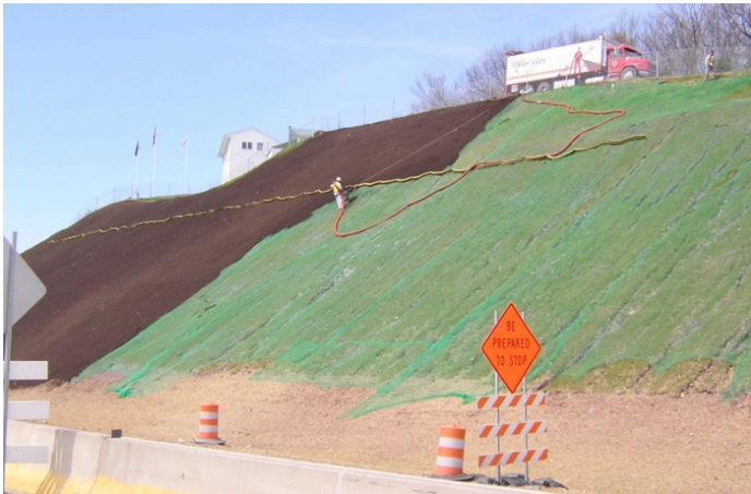
Figure 6. Applying a compost blanket in PA (photo credit: D. Caldwell)
