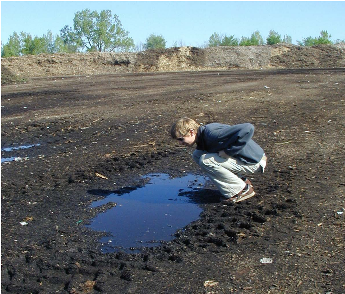
Problem: Anaerobic smell. Cause: Water pooling on compost pad. Solution: Restore grade and repair pad to remove low spots that allow water to puddle.
