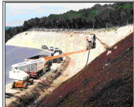
Application of a 2 inch-thick compost blanket to a 1:1 rock slope using a pneumatic blower (Austin, Texas, 2002). Source: McCoy, Texas Commission on Environmental Quality (TECQ), 2005
