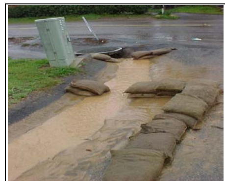
Poorly maintained BMPs can result in significant quantities of sediment being discharged to storm drains.
