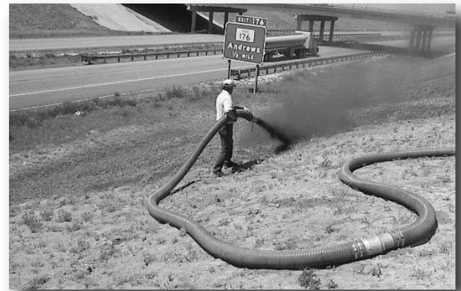
Figure 2 – Applying Compost
