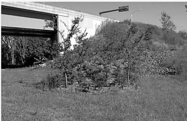
Figure 1 – I-91/Route 3 Interchange Plantings
